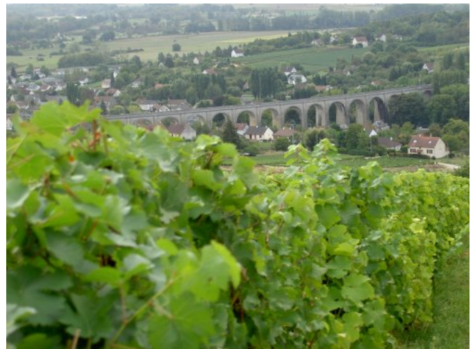
Viaduct of Saint Satur
